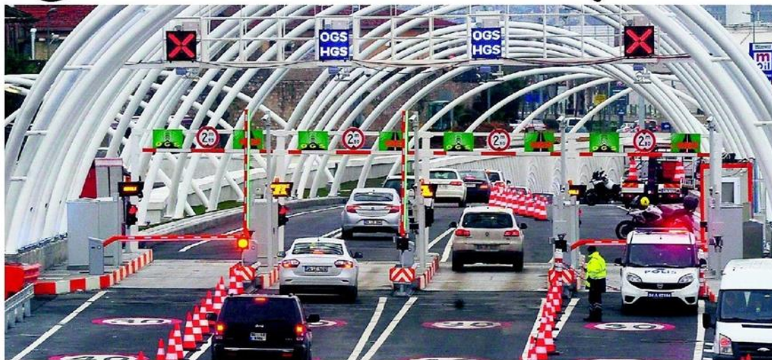
The Eurasia Tunnel was constructed in partnership between Turkey's Yapı Merkezi and SK E&C of South Korea, with an estimated $1.25 billion investment.
