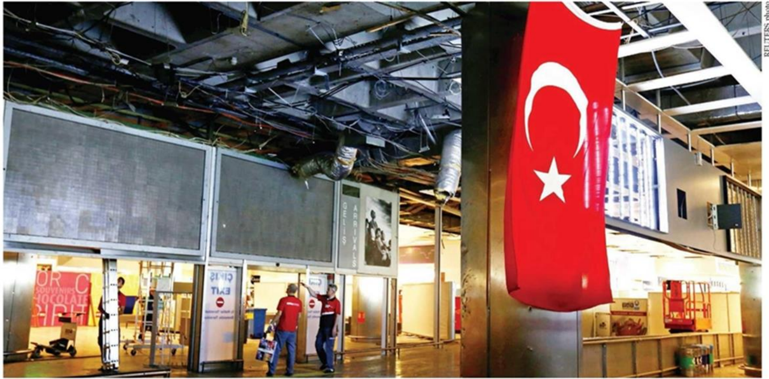
Workers repair the damaged parts of the terminal building at Turkey's largest airport, Istanbul Atatürk, following a number of blasts by suspected Islamic State of Iraq and the Levant (ISIL) militants.
