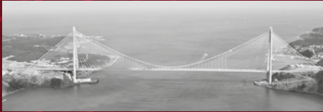
Yavuz Sultan Selim Bridge & North Marmara Motorway, Turkey
