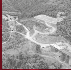
Zenica North Motorway, Bosnia & Herzegovina
