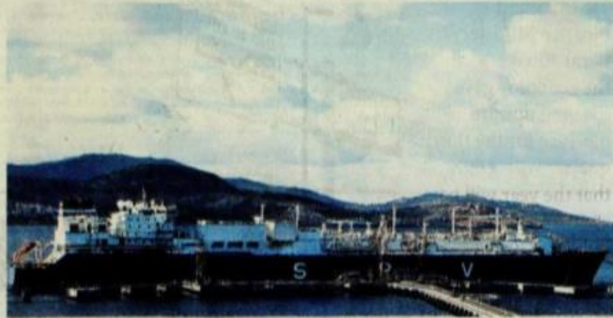
GDF Suez Neptune, a floating storage regasification facility (FSRU) that is among Turkey's LNG investments made in recent years, seen docked in the Aliaga district of western Izmir province, Turkey, Dec. 15, 2016.
