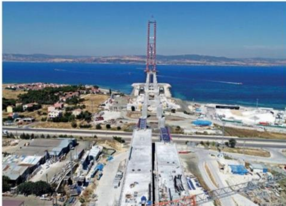
Turkey on May 16 completed 32 tower blocks of the 1915 Çanakkale Bridge, which will be put into service on March 18, 2022. DHA photo
